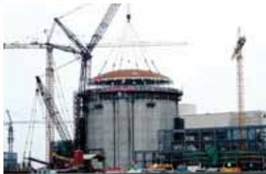
Figure 4: Very-heavy-lift crane and open-top, modular construction at Qinshan Phase III, China
